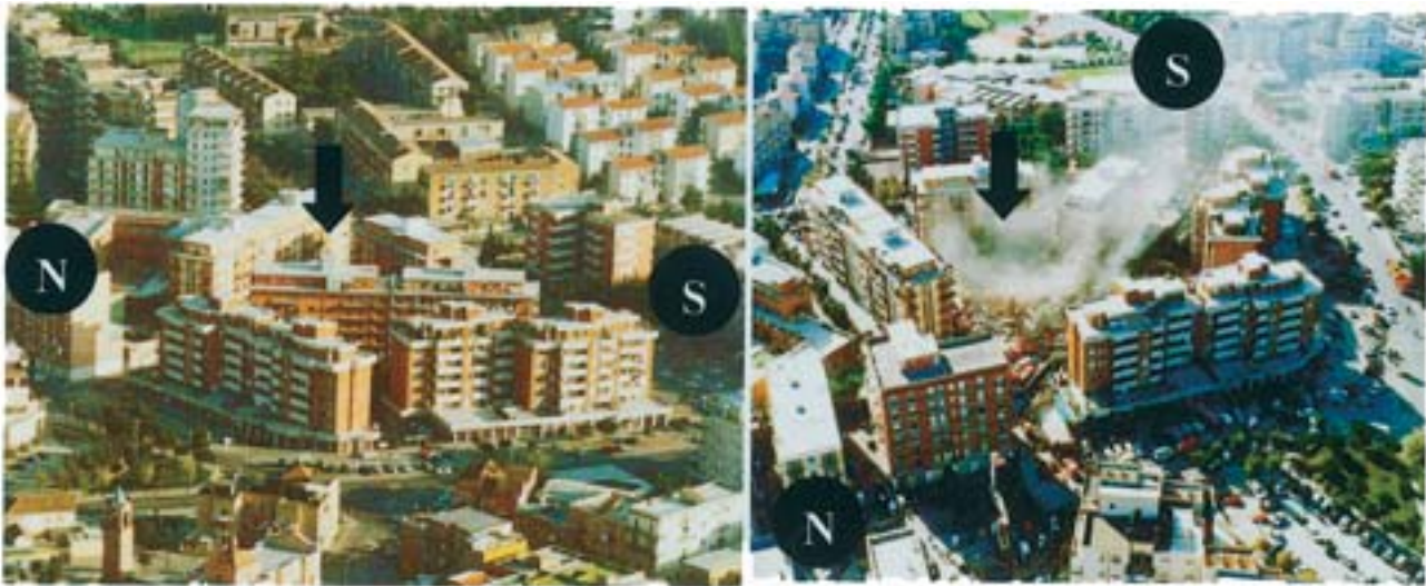
FIG. 1—Aerial view of the six-story apartment building before and after the collapse.
